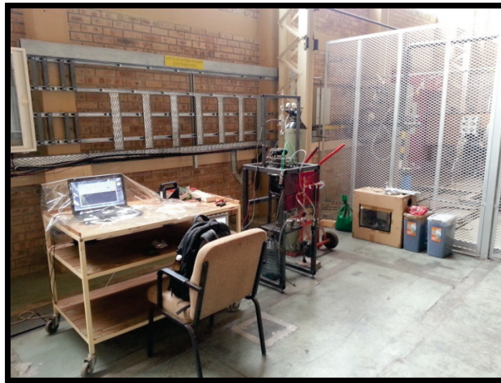
Figure 38: PF feeder moved indoors.
