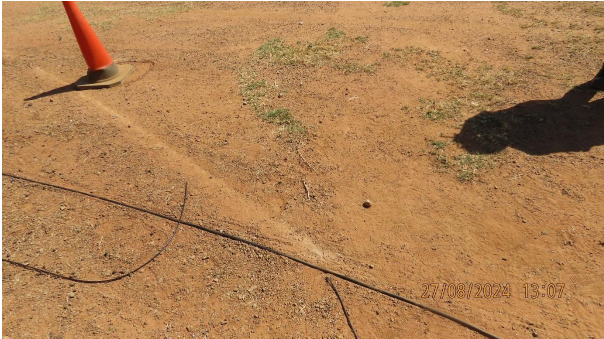
Figure 52: Damaged BNC cable
