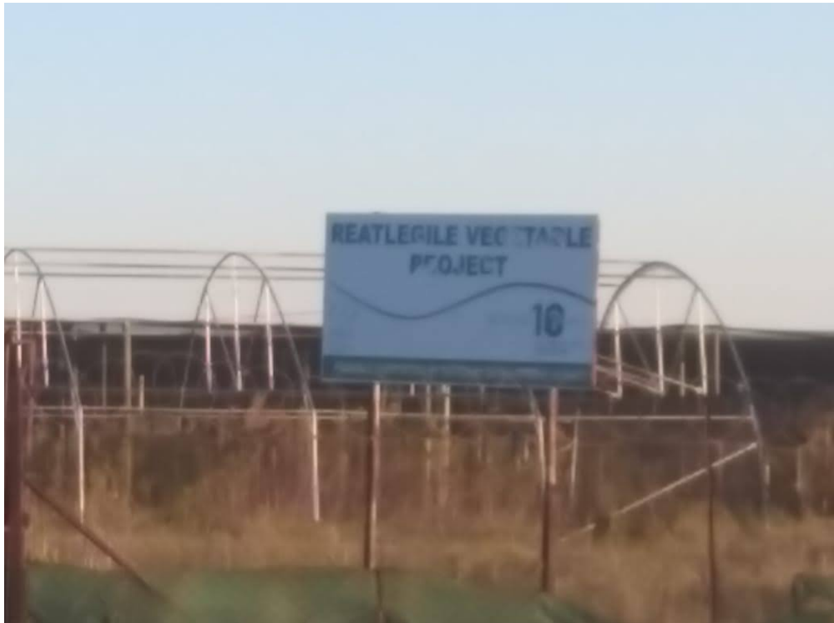
Figure 5.2 (b): CPA with infrastructure that is not well-maintained.
