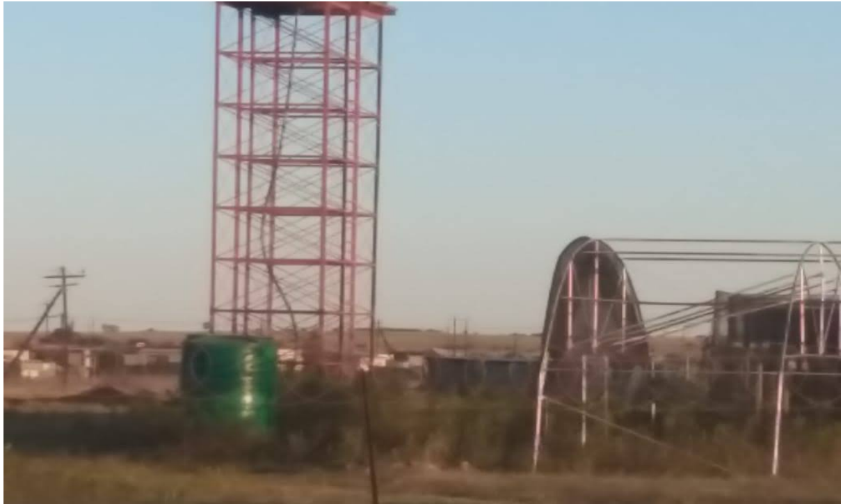
Figure 5.2 (a): CPA with infrastructure that is not well-maintained.
