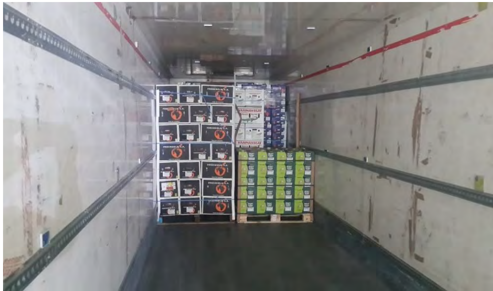
Figure 3-10: Inside a trailer showing installed sensors on sides
