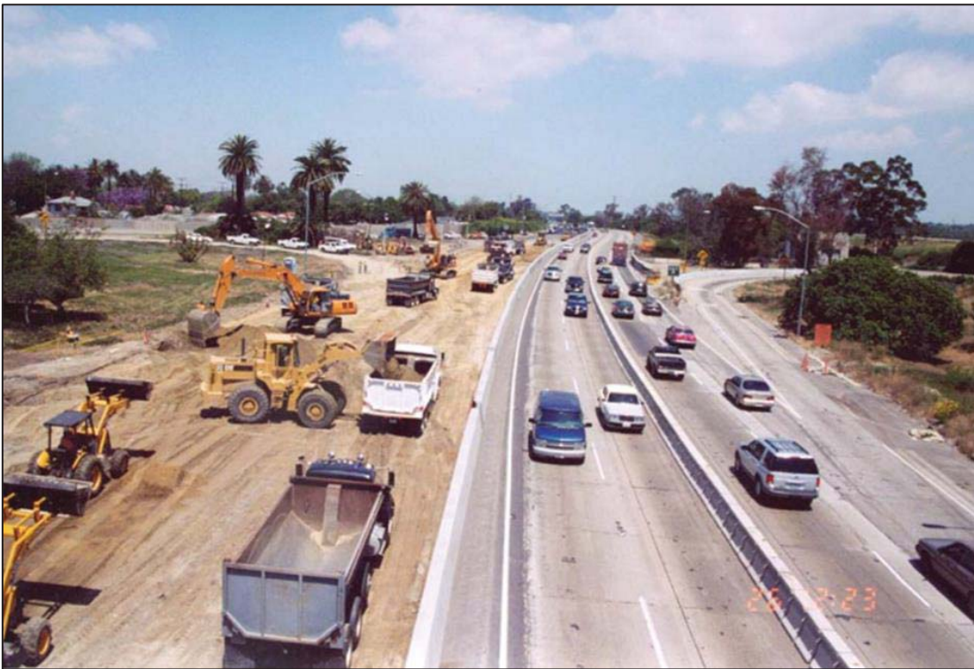
The I-710 rehabilitation construction during a 55-hour weekend closure
