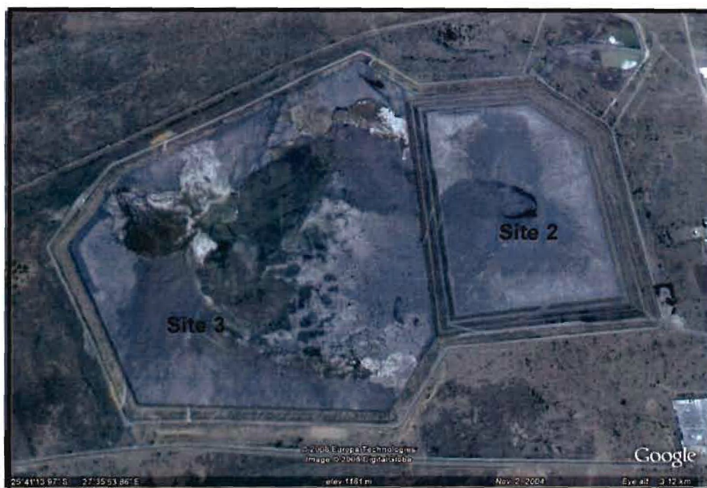
Figure 5. Aerial photograph of site 2 and site 3, prior to rehabilitation of site 2 (Google Earth, 2008). The dark colours of the materials are attributed to the high chrome content of the UG2 reef.
