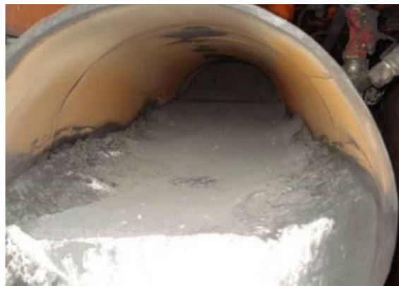
FIGURE 2.8: PF SETTLING IN A BURNER PIPE (van der Merwe, 2014:10)
