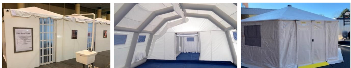
Figure 4.2 Examples of temporary facilities: Rigid-type building, inflatable tent-type and framed tent
