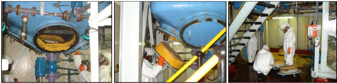
Figure C6. Bay 3 . Removing module filters (2.507 g/m 3 )
