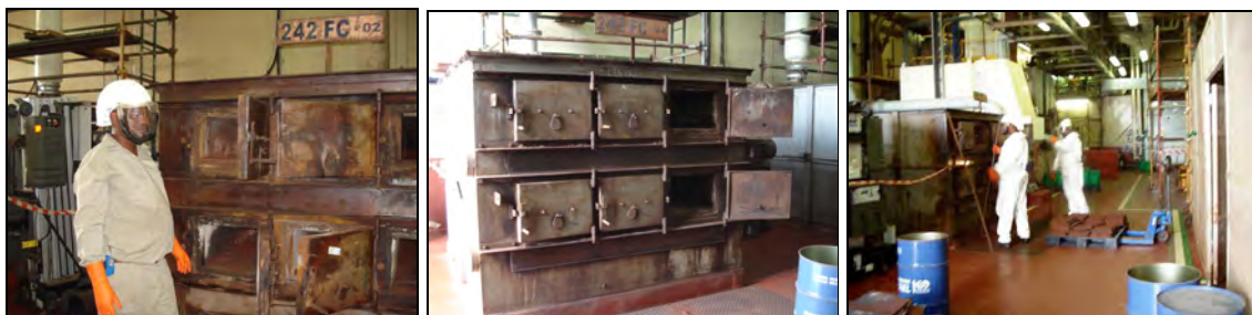
Figure C3. Bay 5 - Dismantling (3.916 g/m 3 ) and cleaning (5.544 g/m 3 ) muffles
