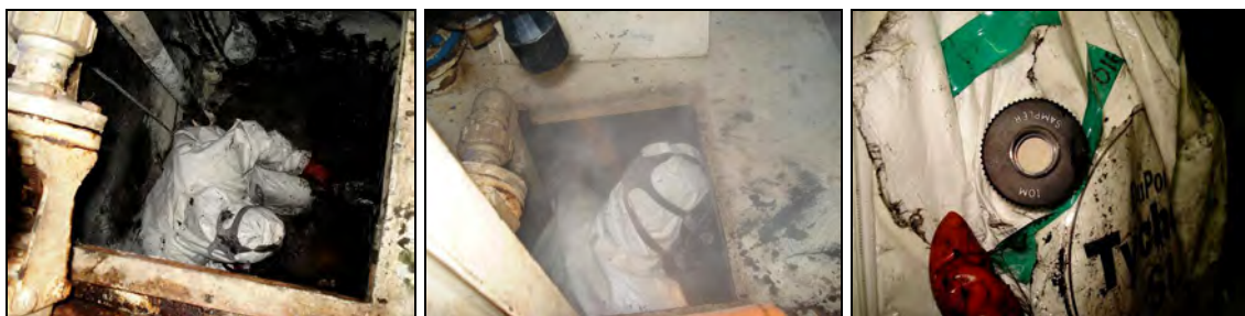
Figure C4. Bay 3 . Digging out sump residues (3.732 g/m 3 )
