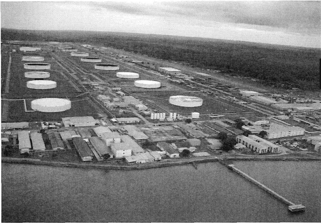
Fig. 5: Arial view of Chevron-Escravos tank farm
