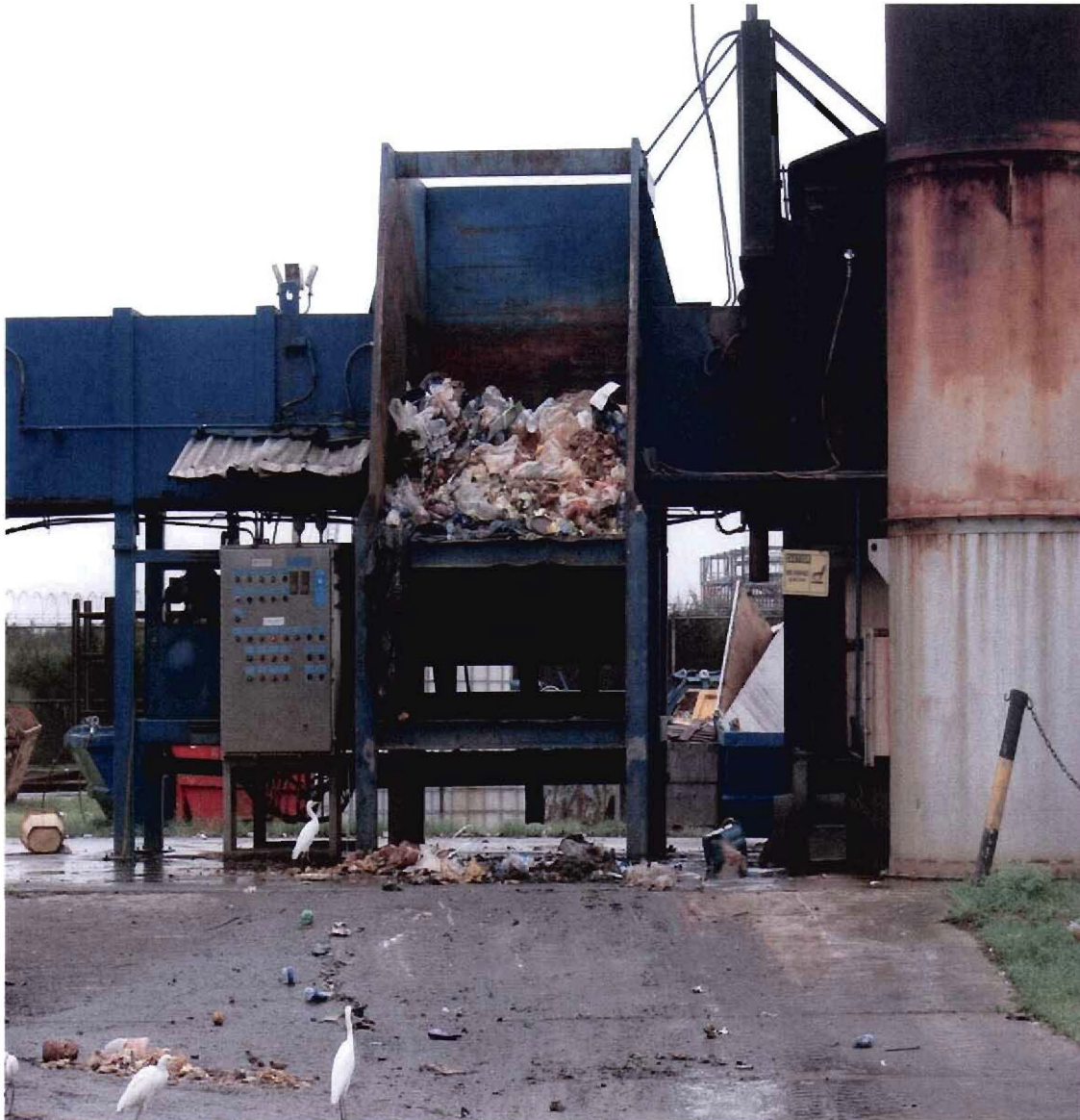
Fig. 7: Chevron-Escravos incinerator, showing organic waste being loaded for combustion.
