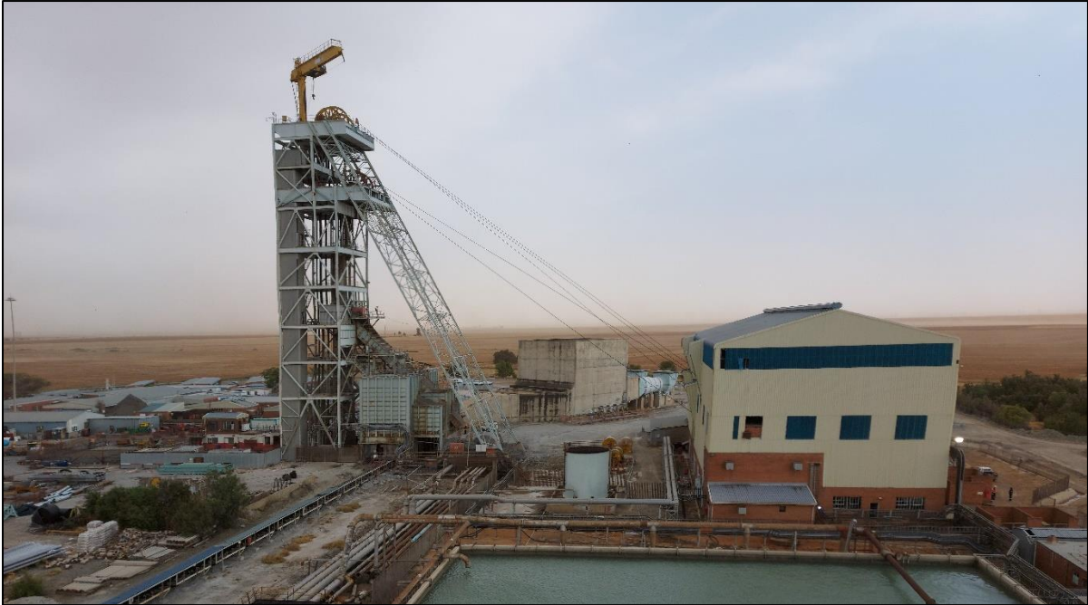
Figure 55: Typical deep-level mine in South Africa 4
