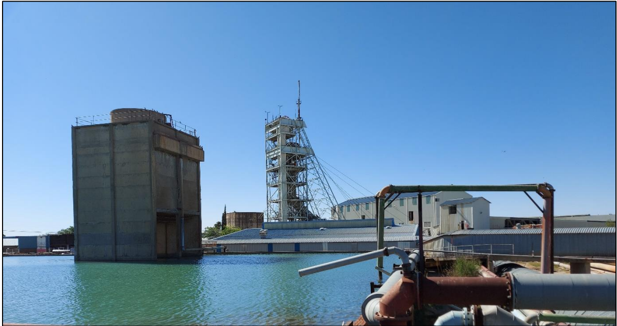
Figure 1: Typical South African mine 1
