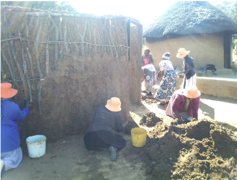
Fig. 11 Community members building rondavels for accommodating visitors project participated by Wits University and Ditsong National Museum of Cultural History
