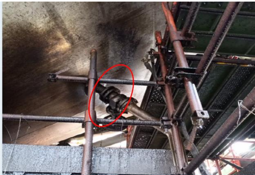
Figure 20: The area where the blank was removed for box-up. The red marking is on the drain line flange. Image used with permission from source that wishes to stay anonymous.
