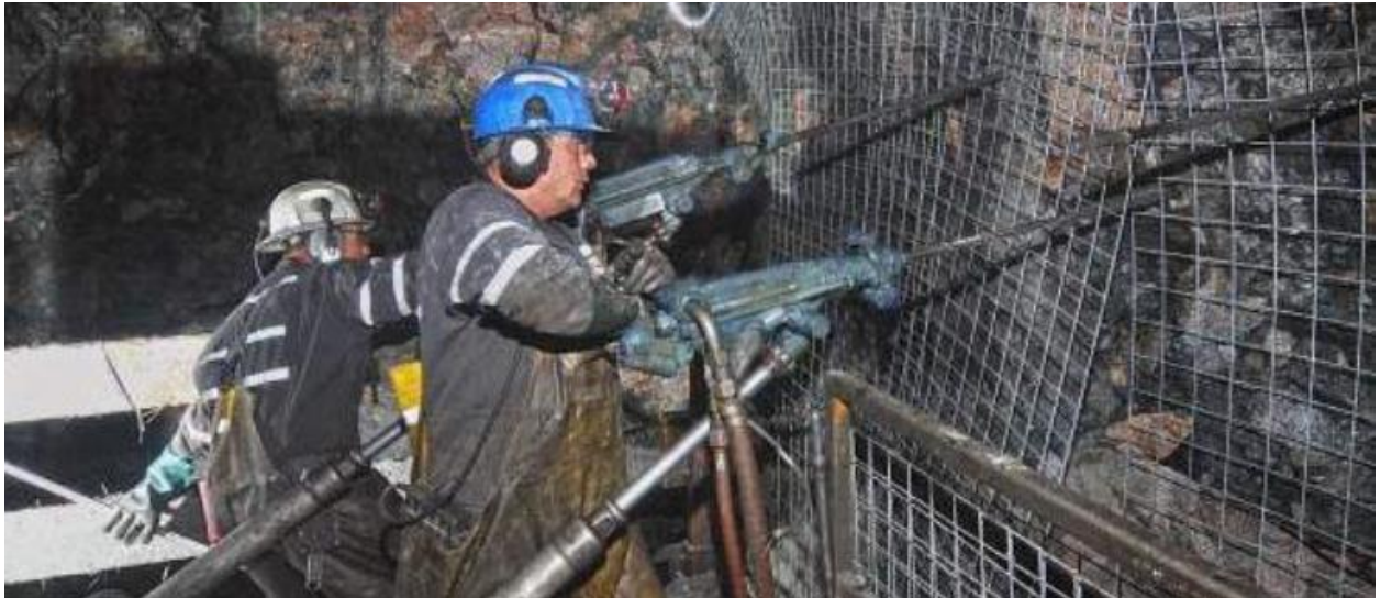
Figure 1-6: Typical rock drill operation [16]
