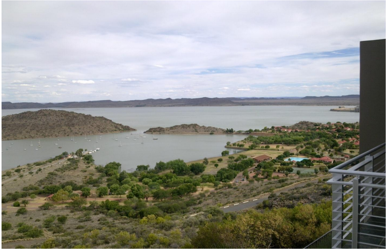
Photograph 2: South Africa's biggest dam (the Gariep) in the Orange River in the Free State Province. Photographer: J De Ridder
