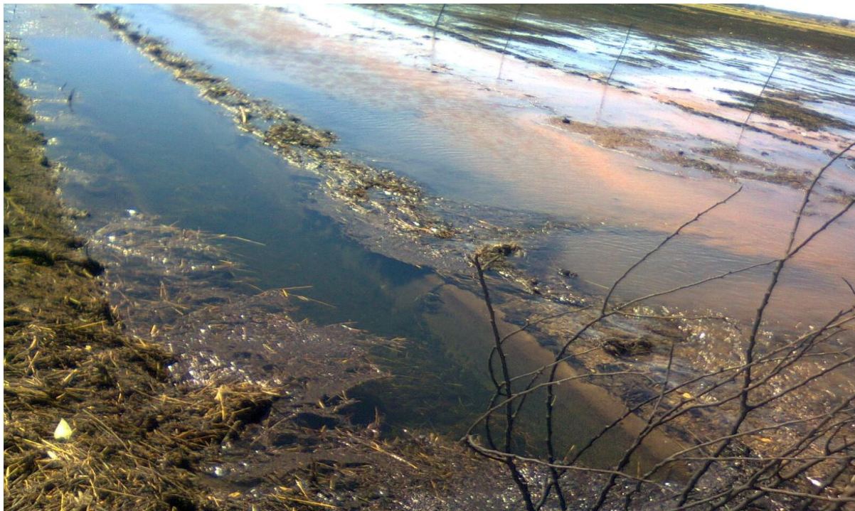
Photograph 1: Canal overflowing due to poor maintenance, Location: Haaskraal, Mooibank Photographer: T Chupeco
