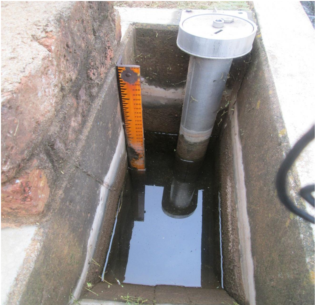
Photograph 6: Dry Mooibank (LRO) canal with a standing gauge
