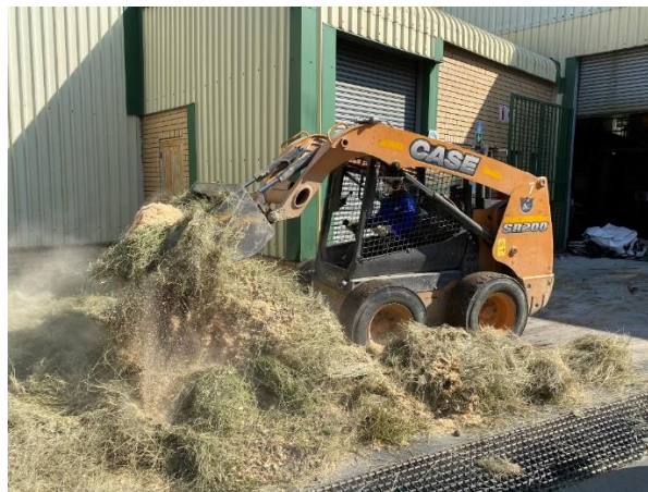
Figure 6. Photograph showing the mixing of the bed material with a skid steer loader
