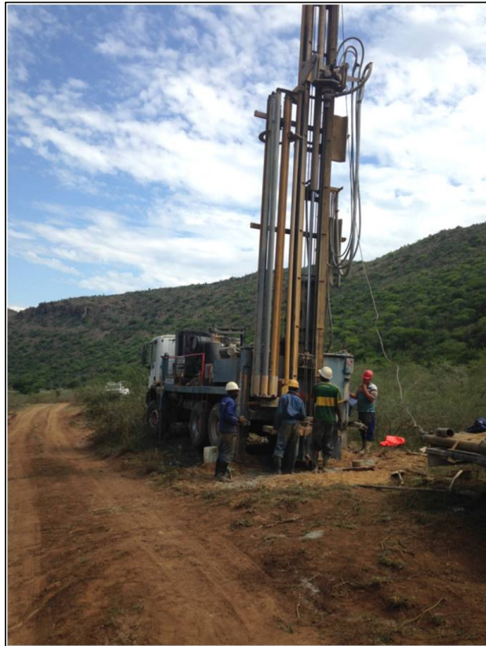
Figure 8 A drilling rig being operated during the study.
