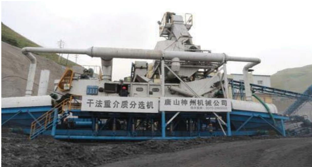
Figure 2.8-1: World's first modularized dry coal beneficiation plant (Zhao et al. , 2016)
