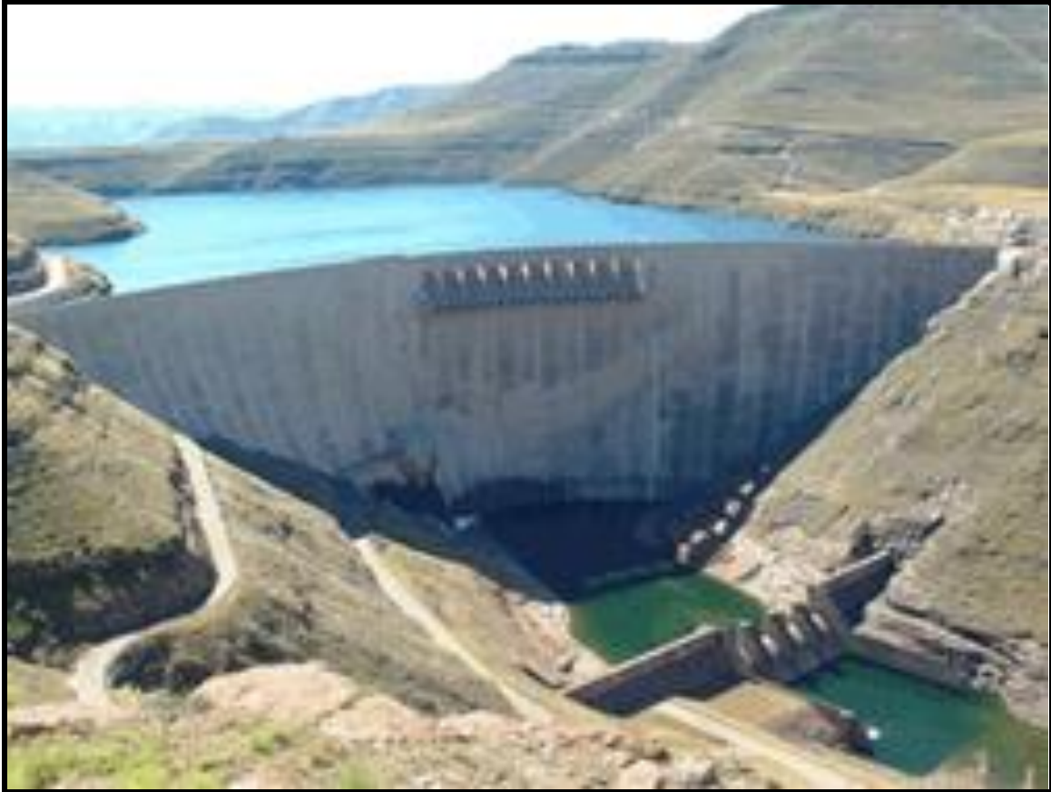
Figure 5.20: The Lesotho Highlands water project
