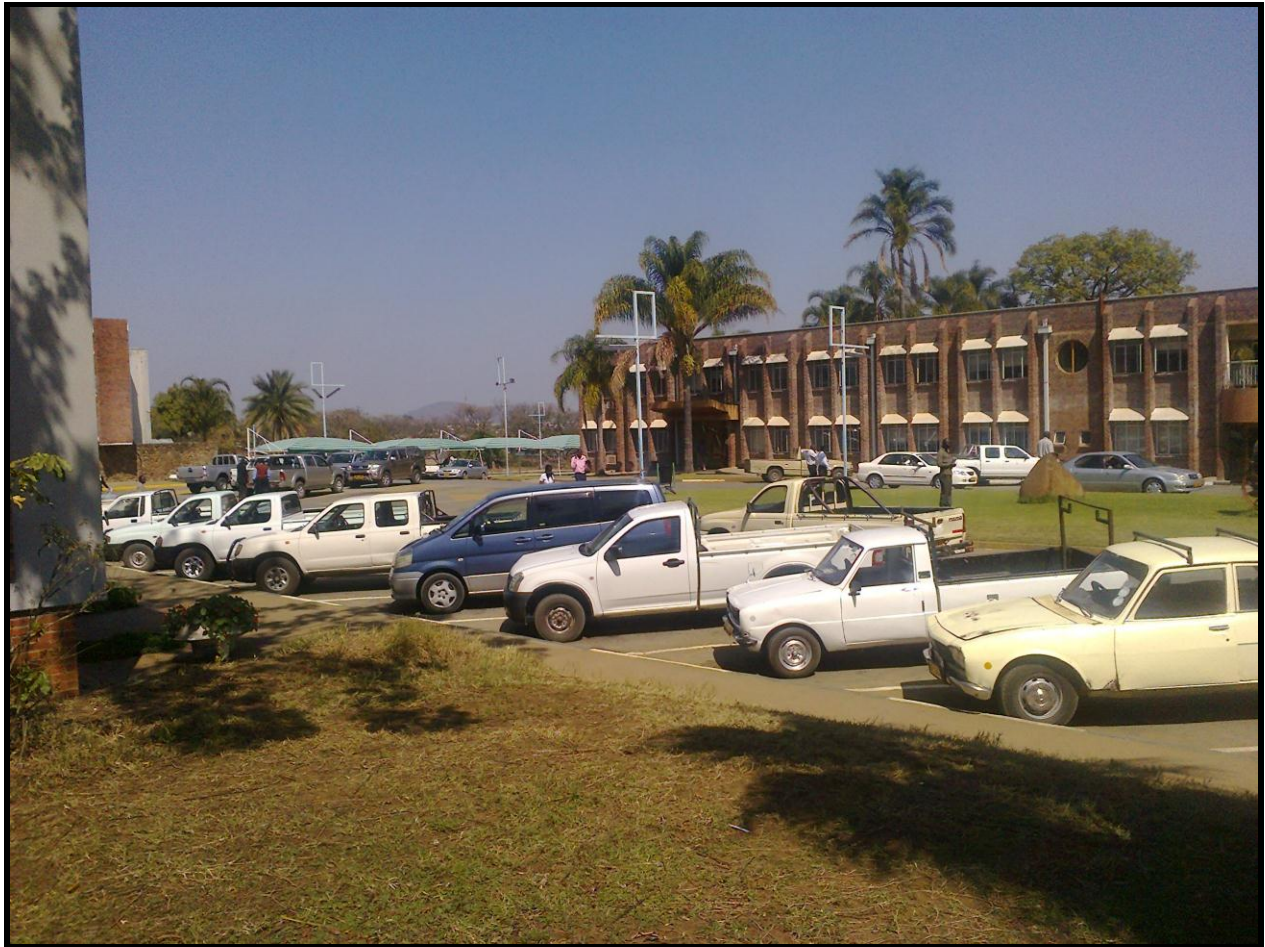
Figure 5.10: Masvingo municipality offices
