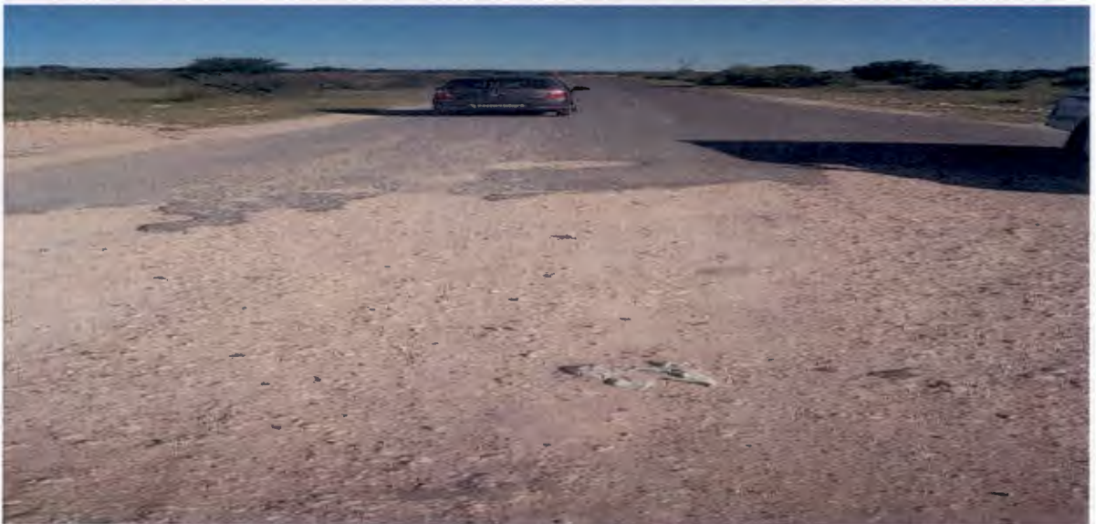
Figure 11: Greater Taung road source: field observation
