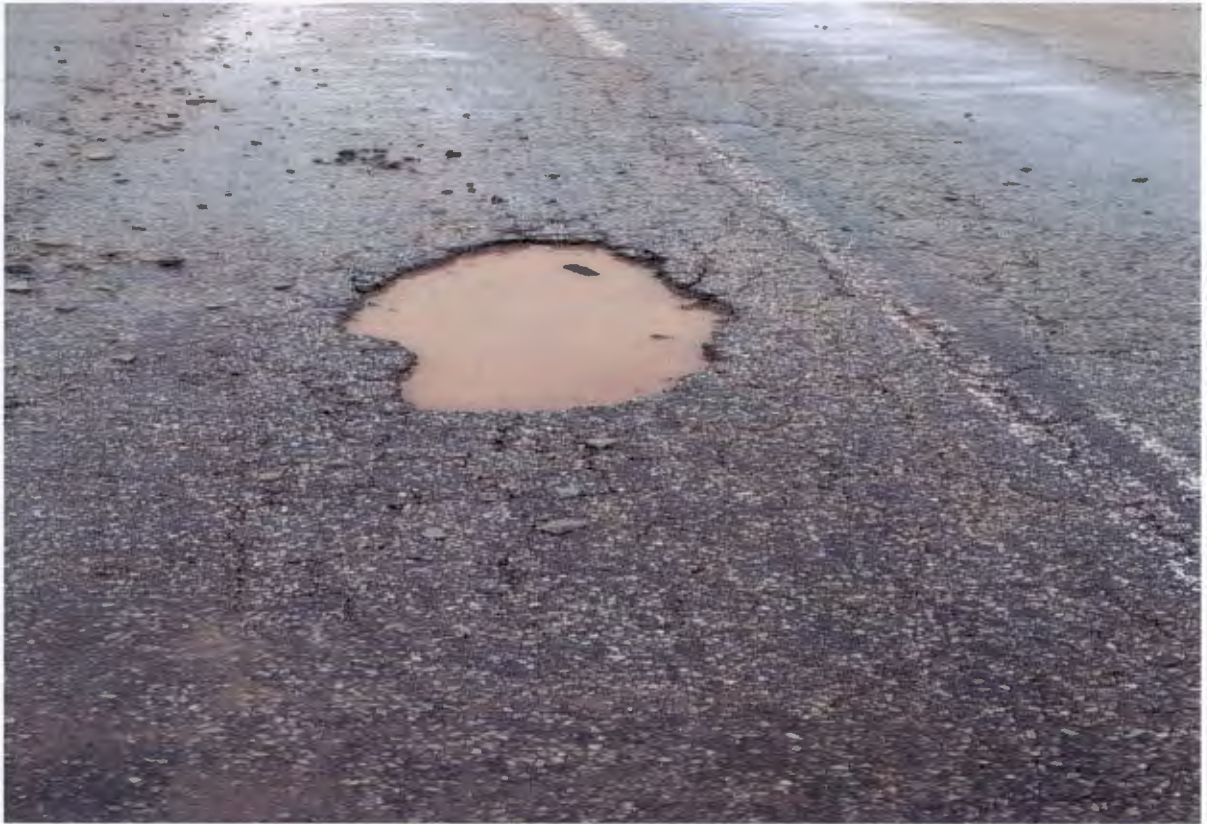
Figure 10: lekwaTeemane road source: field observation
