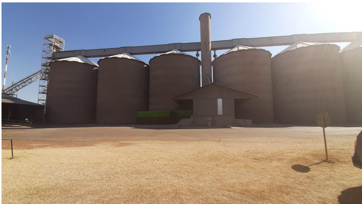
Figure 18: Photograph of the Grootpan silo
