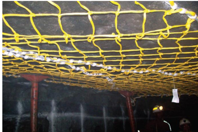
Figure 13: Mechanical jacks used to clamp braided mesh to the hanging wall (Skarbøvig et al. , 2011)
