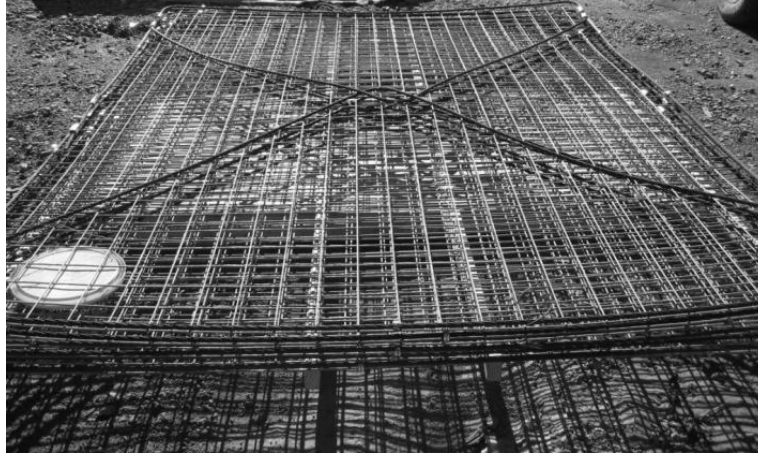
Figure 11: Welded mesh reinforced with wire rope (Potvin and Heal, 2010)
