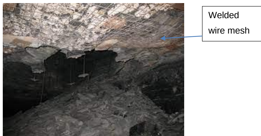
Figure 1: Welded wire mesh installed underground
