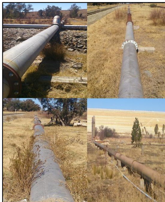
Figure 82: Interconnecting pipeline installed to export compressed air from 1# to 2# 16
