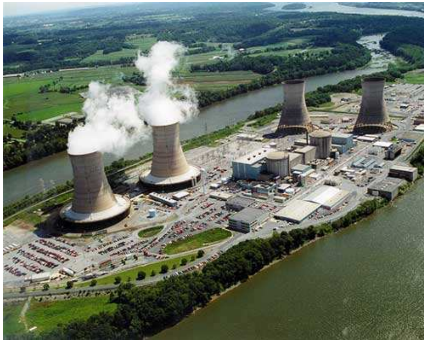
Figure 49: Three Mile Island nuclear power plant (Source: http://thenewschronicle.com )
