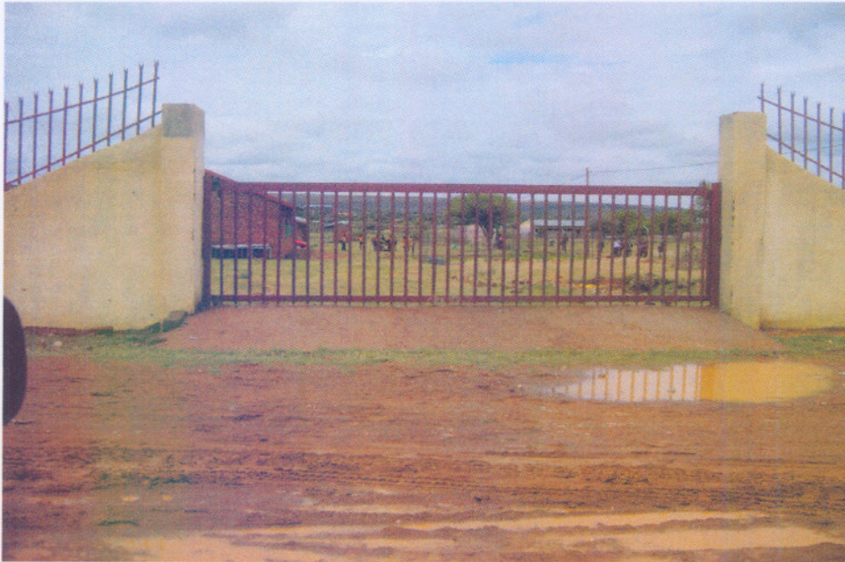
Figure 4.5A A secure school perimeter fence and gate
