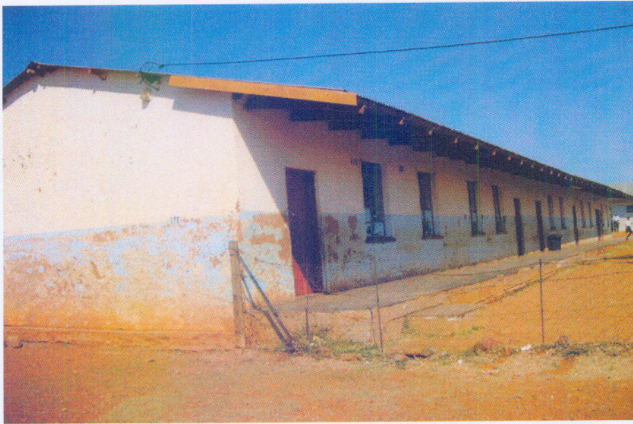
Figure 4.1A The Cosmos High school buildings
