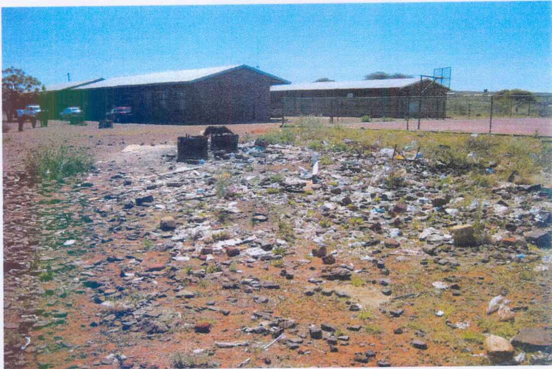
Figure 4.20: Open refuse dumps
