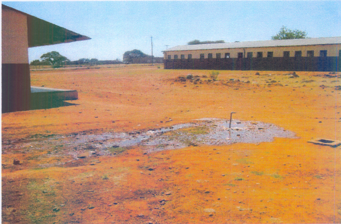
Figure 4.19: Stagnant water around a tap stand
