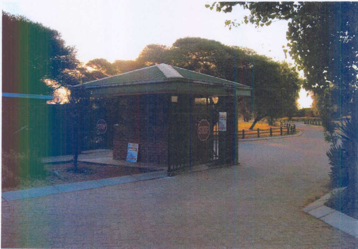
Figure 4.6B: A secure school gate and security office
