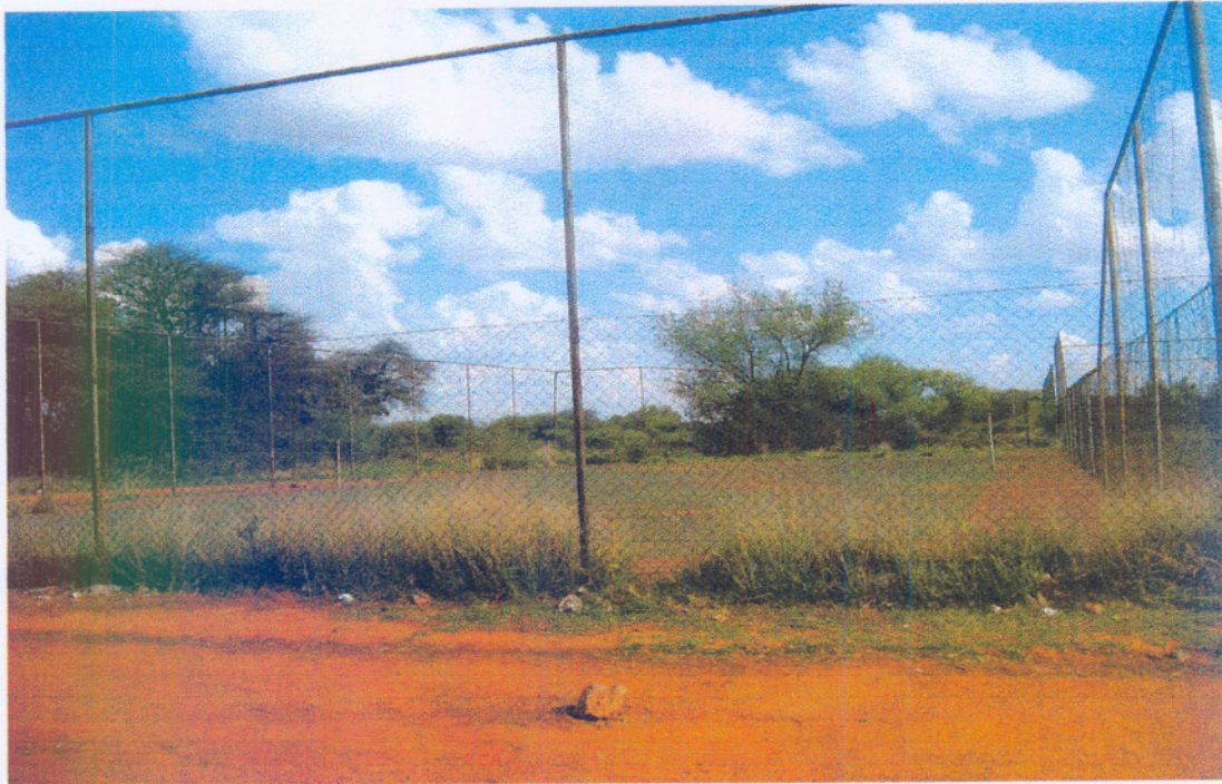
Figure 4.9: Poorly maintained tennis courts
