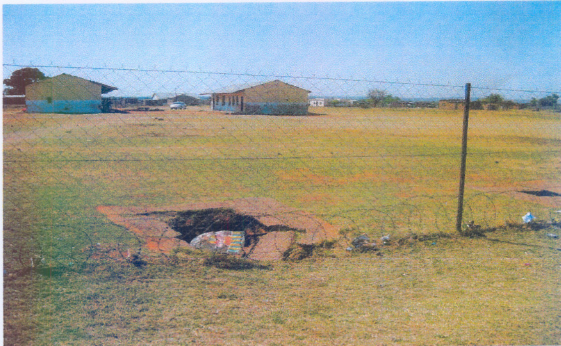
Figure 4.22: An unmarked safety hazard
