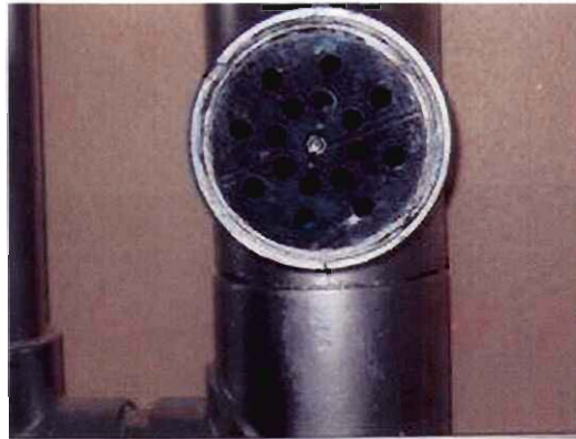
Figure 4. 11: Close-up view of an individual air nozzle, designed to allow uniform air movement across each guinea pig cage
