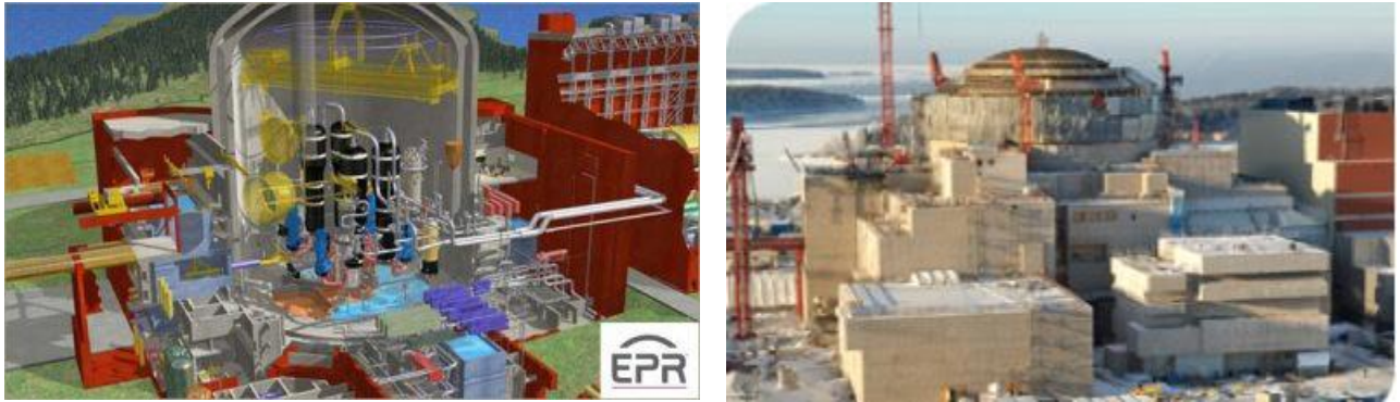
Figure 2-6: EPR plant layout and plant under construction in Okiluoto
