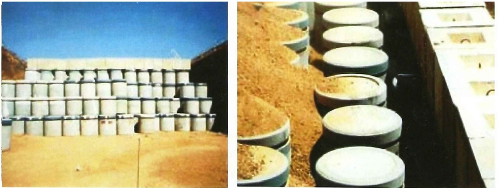
Figure 1.2(A): Cross-sectional diagram of waste disposal at Vaalputs showing the placing of cement drums in trenches before filling the trench and covering it with clay.
