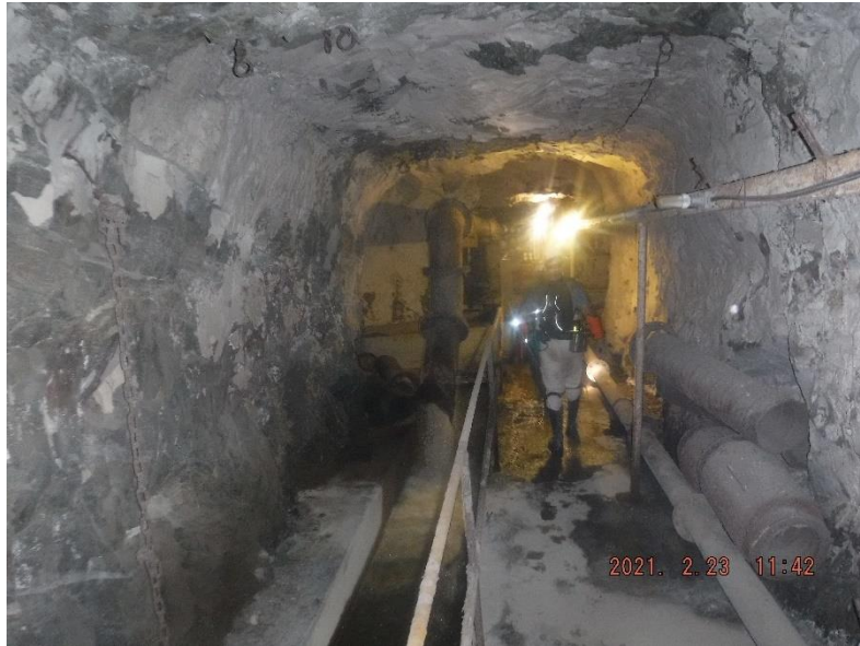
Figure 70: Dewatering pipe opening into a drain in the settler area
