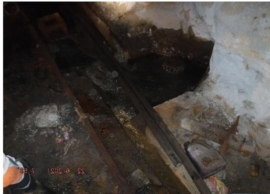
Figure 56: Mine drain hole
