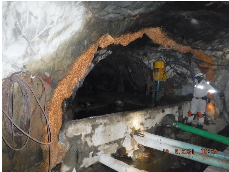
Figure 48: 24L cofferdam area
