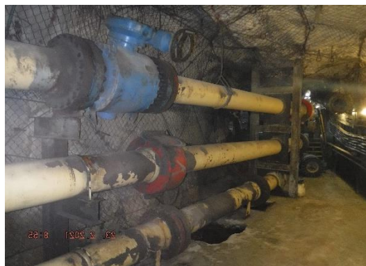
Figure 54: Three underground dewatering pipes
