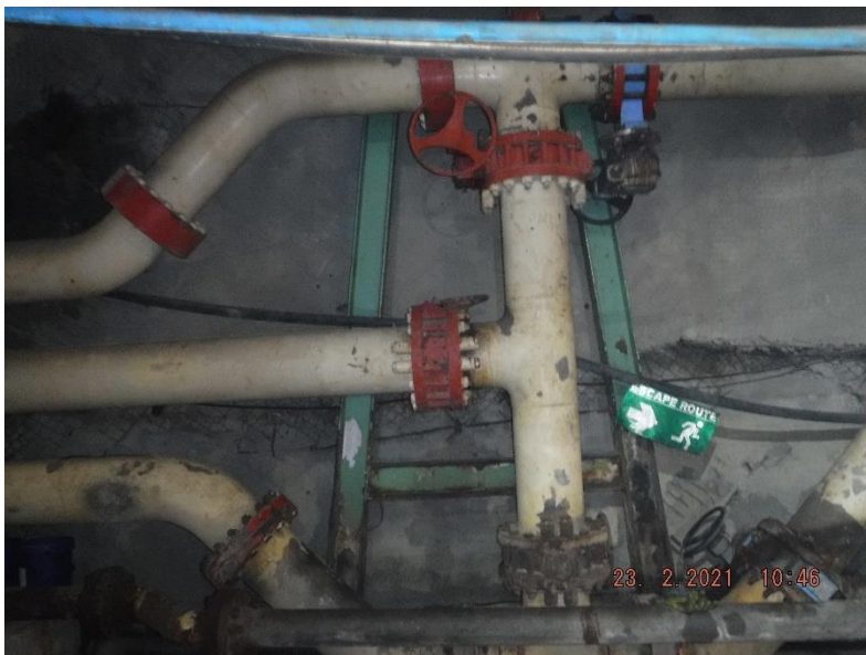
Figure 69: Dewatering pipe configuration with valves
