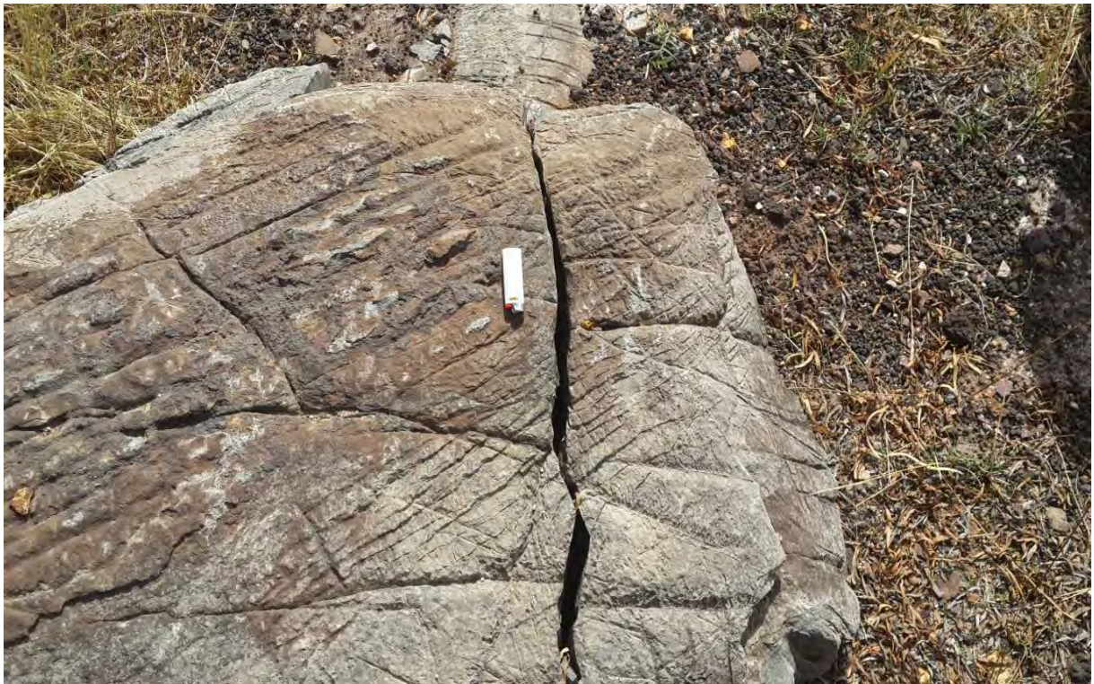
Figure 5: Joints and fractures present in, and on the surface of, the Oaktree Formation dolomites. Photograph taken by Daniell (2013).
