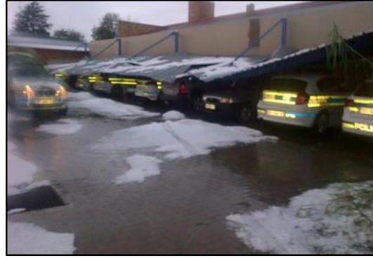
Figure 2-8: Illustrates a collapsed roof on vehicles prior to the hail event.
