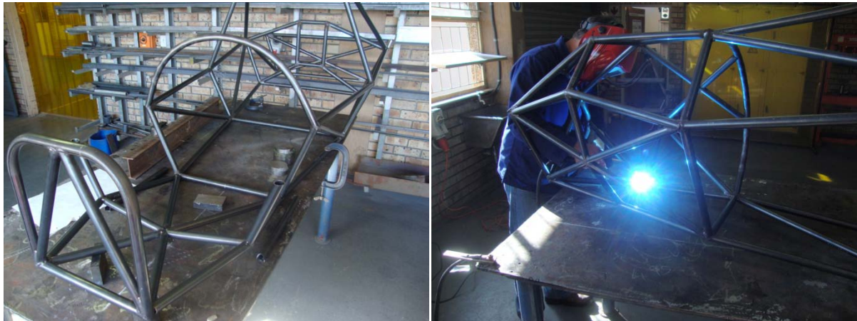
Figure 5-17: Photos of the front structure under construction
