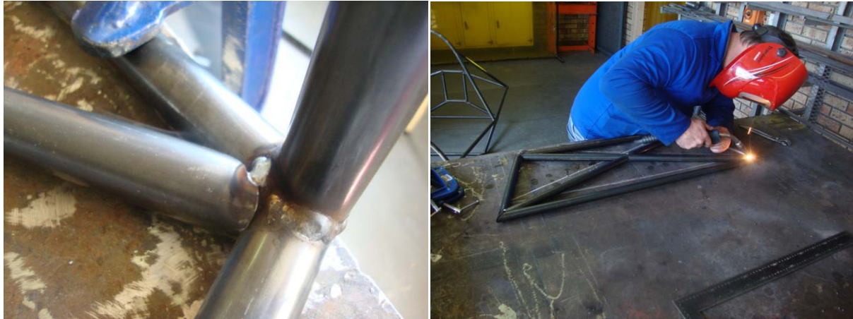
Figure 5-16: Photos of a tack welded joint (left) and a structure undergoing tack welding
