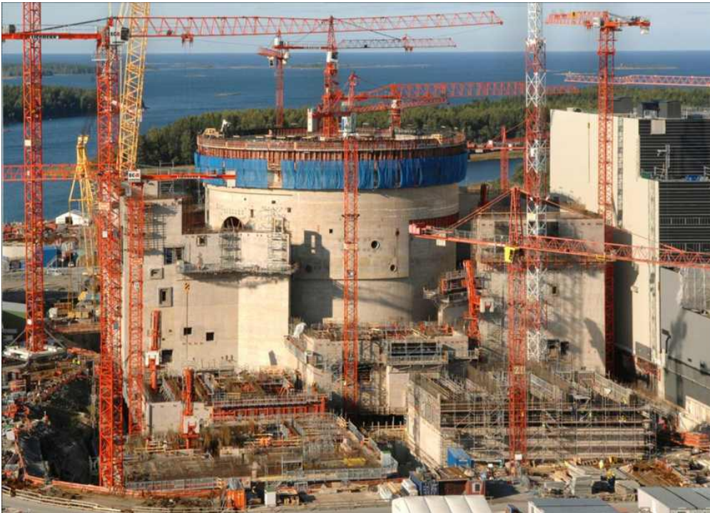
Figure 3-2: Olkiluoto U3 NPP Construction Site (Source by Areva)
