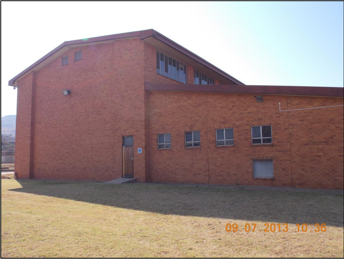
Figure 93: Engine Room from the outside
