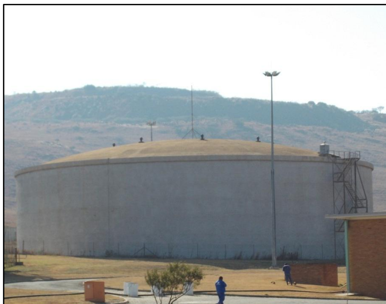
Figure 22: On-site demand-balancing reservoir part of the integrated WDU
