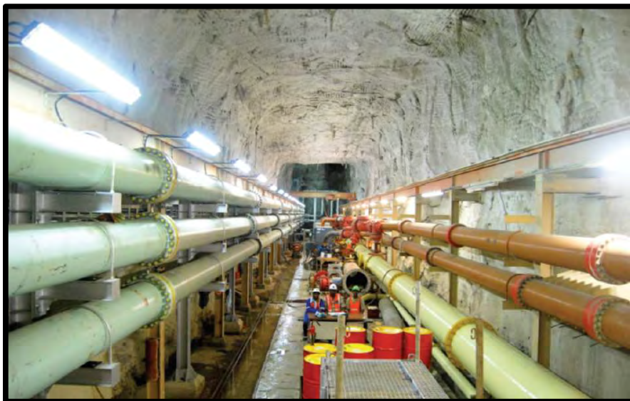
Figure 28: 3CPFS hydro-lift chamber excavated space and pipes
