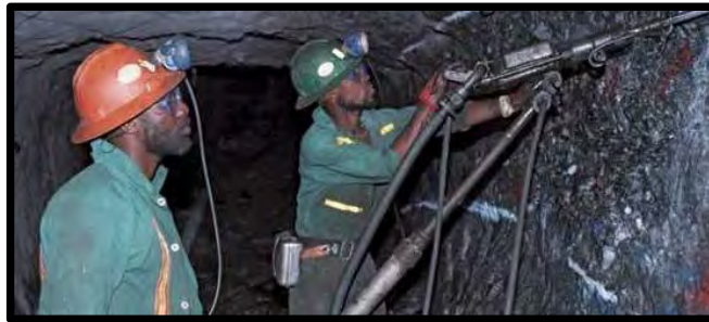
Figure 31: Miners drilling holes with hydro-power equipment
