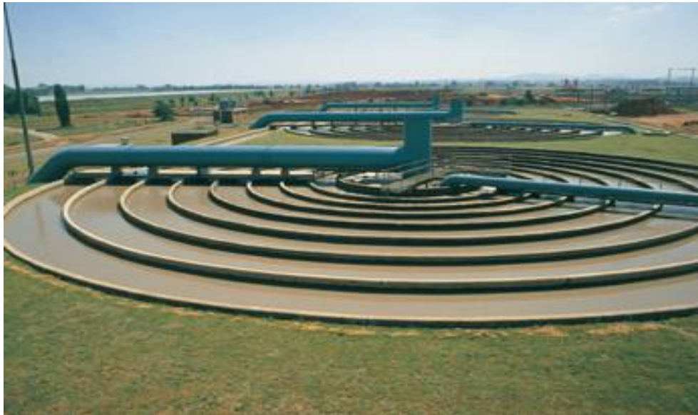
Figure 6: Flocculation process in conventional water treatment plants
