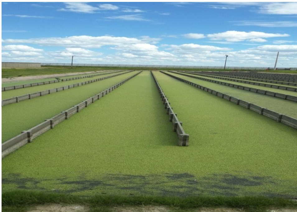
Figure 1-6: Evaporation pond on the sewage plant situated in Bethal, South Africa
