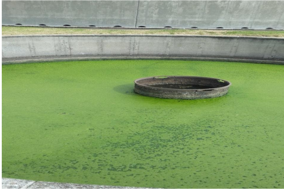
Figure 1-5: Open pond on Sewage plant situated in Bethal, South Africa
