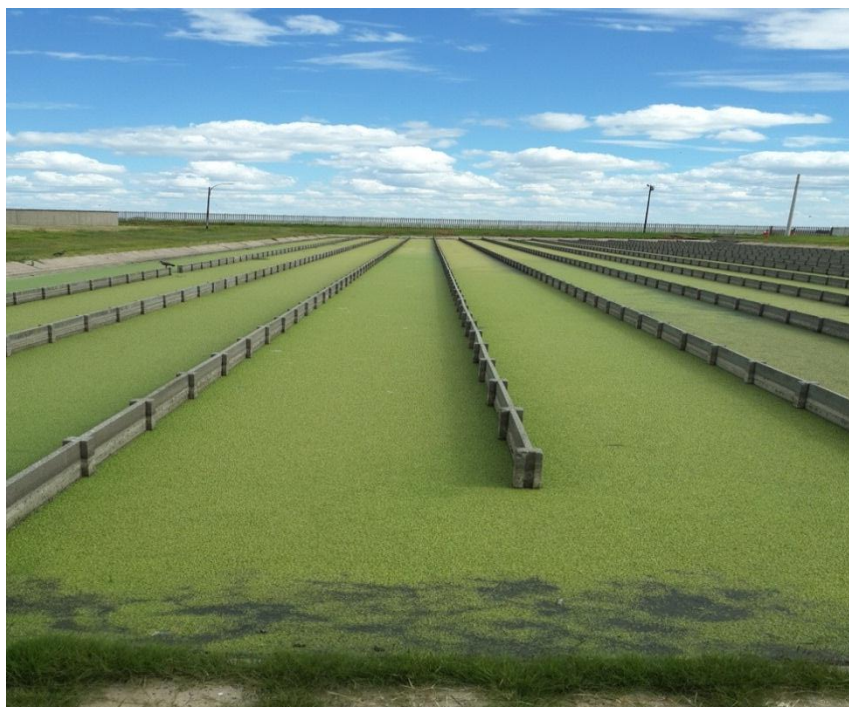
Figure 3-1: Evaporation pond at the sewage plant situated in Bethal, South Africa
