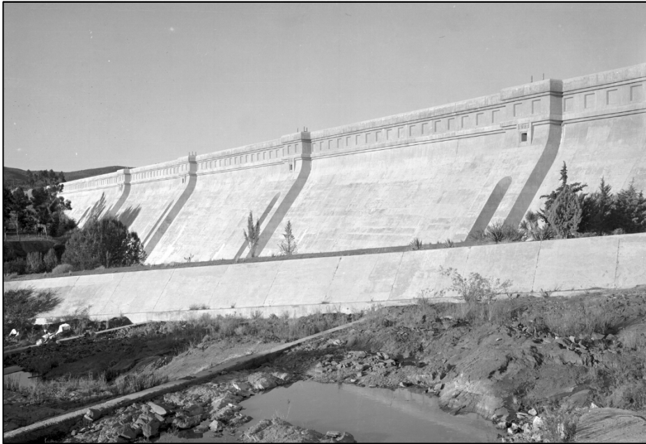
Figure 3-2: Kamanassie Dam outside Oudtshoorn, constructed between 1919 and 1925 87
