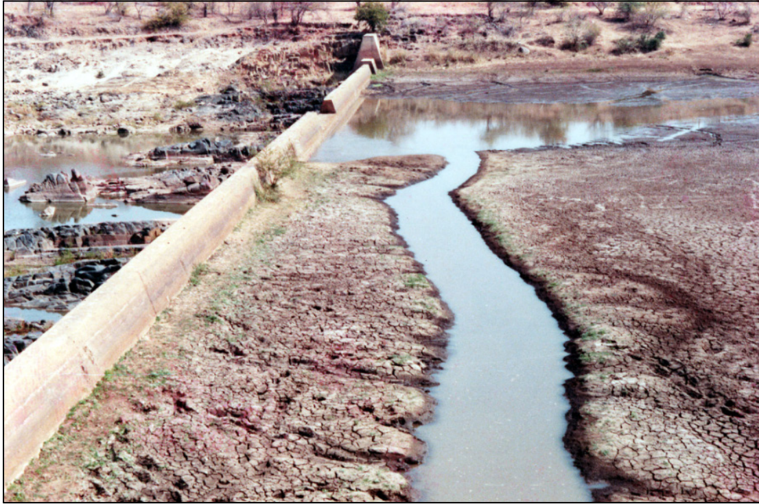
Figure 5-5: Black Heron weir – constructed in the Letaba river inside the Kruger National Park – had completely silted up by 1986. It has since been converted into a measuring weir 109
