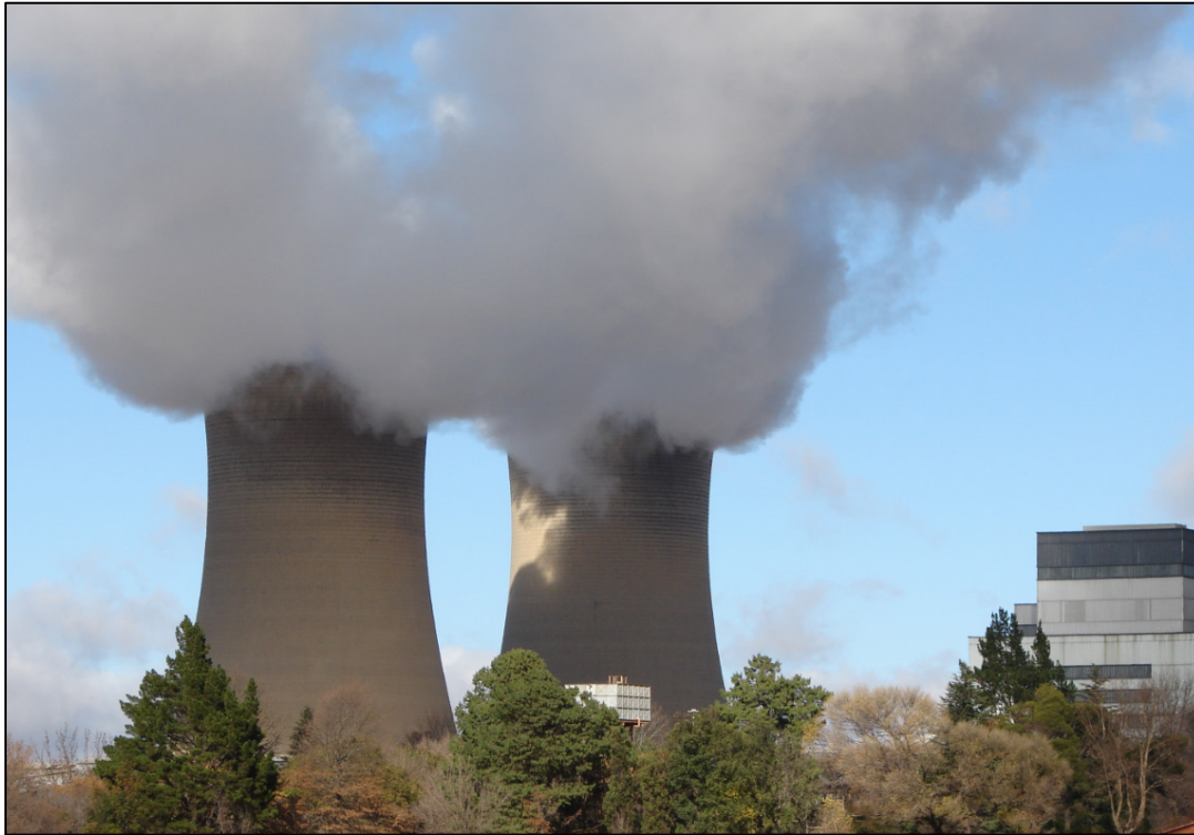
Figure 2-13: Kriel Power Station, one of eight power stations that have been developed in the Upper Olifants River catchment 112
