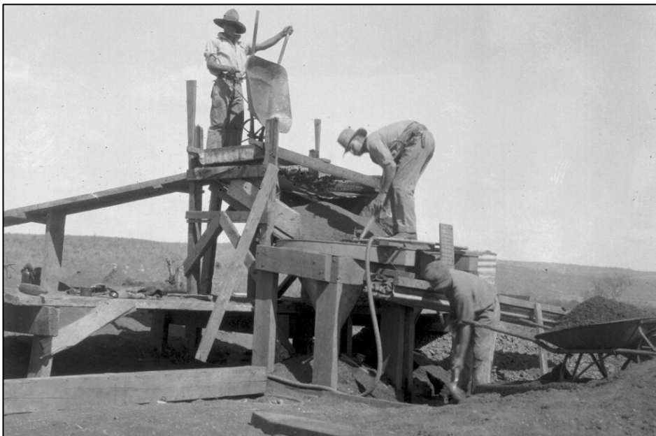
Figure 3-3: Workers washing sand on the Marico-Bosveld irrigation scheme construction site in 1932 88
