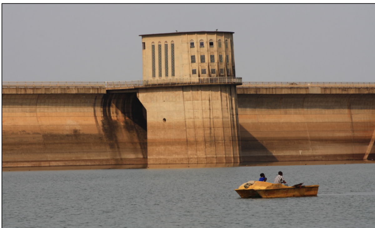
Figure 4-2: The Pongolapoort Dam wall outside Jozini, Kwazulu-Natal 112
