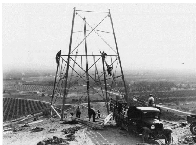
Figure 18 : Construction of a self-supporting structure with a Derek crane
