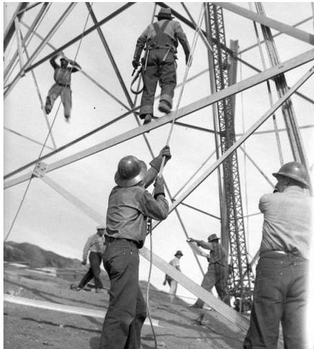
Figure 17: Construction of a self-supporting structure with a Derek crane - Hoover Dam construction (1931-1936)
