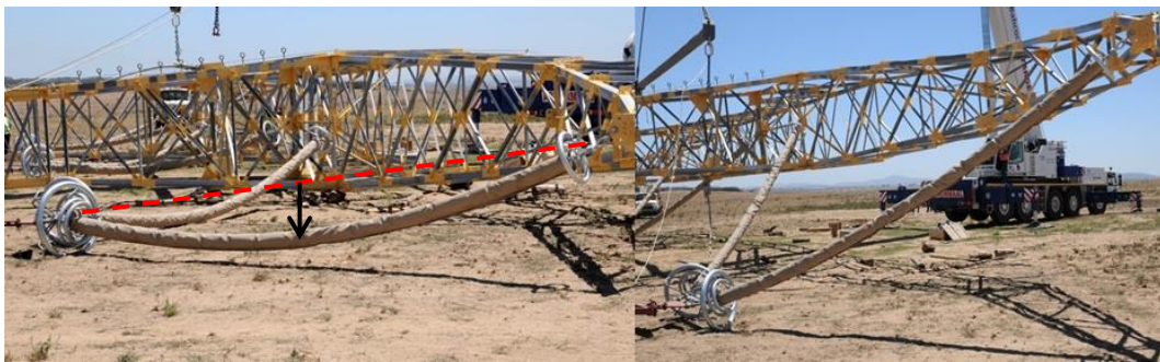
Figure 45: Bending of composite insulator during erection of a guyed-V suspension structure
