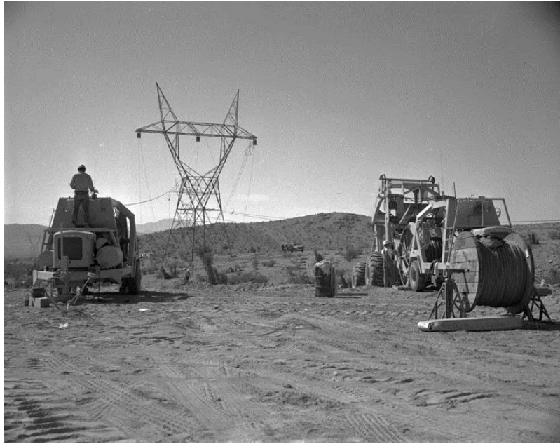
Figure 61: Stringing of Boulder transmission line (266 miles) near Victorville in 1969
