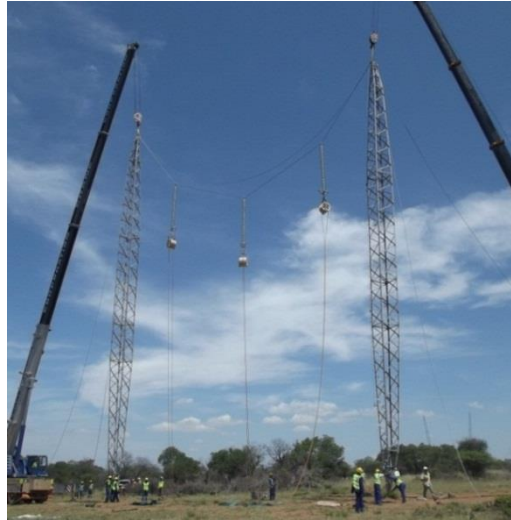
Figure 48: Erection of a guayed cross-rope suspension structure with two cranes
