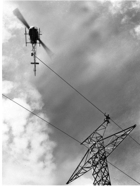
Figure 63: Pulling pilot cable with helicopter on the Pacific Intertie line in 1968
