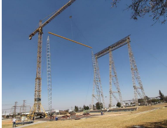
Figure 49: Erection of guyed cross-rope suspension structure with a spreader beam
