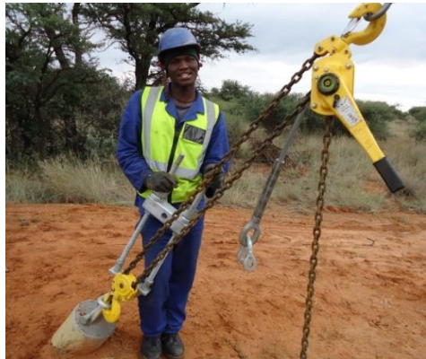
Figure 13: Guy wire during installation with a lever hoist and load cell
