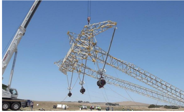
Figure 44: Erection of a guyed-V suspension structure with all accessories
