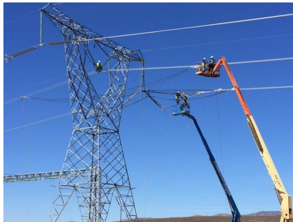
Figure 21: Local use of a cherry picker to install custom assemblies
