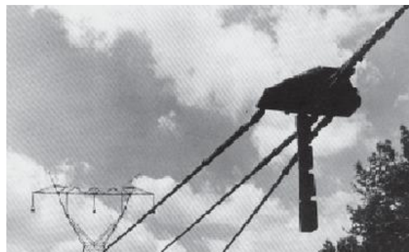
Figure 62: Stringing running board
