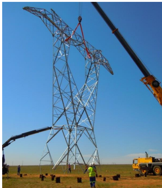
Figure 51: Example of a self-supporting suspension body, K-frames and beam being lifted
