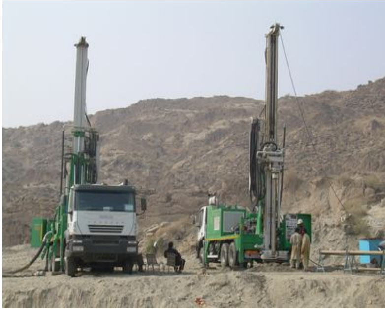
Illustration13: Drilling for water is a long-term solution to communities with no potable water connectivity. Source: the connector drilling.com.
