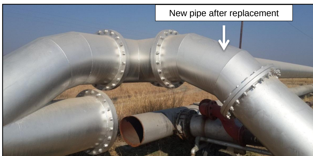
Figure 38: Pipe diameter after replacing the pipe to the shaft
