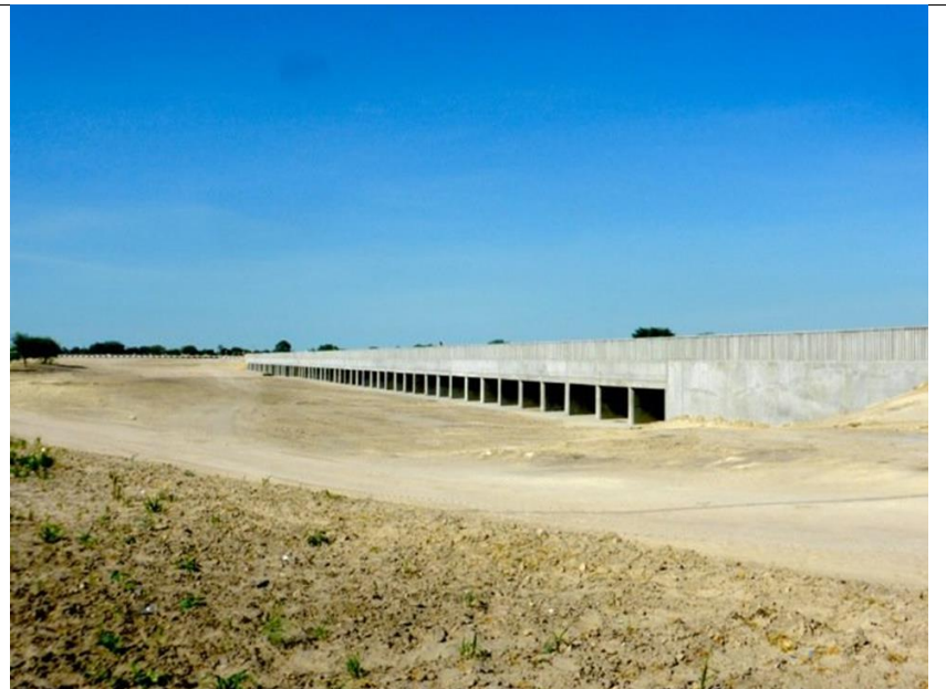
Figure 5.1 Embankment Source: https://imdc.be/en/reference/oshakati-flood-protection
