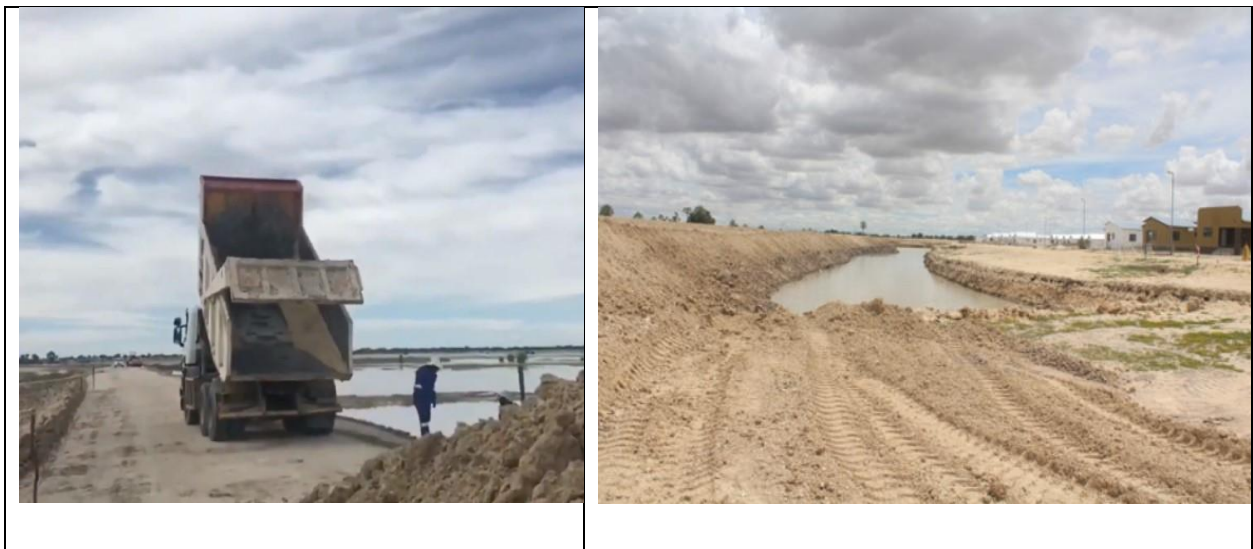
Figure 4. 10 (a) and (b): Ongoing construction of the embankment.
