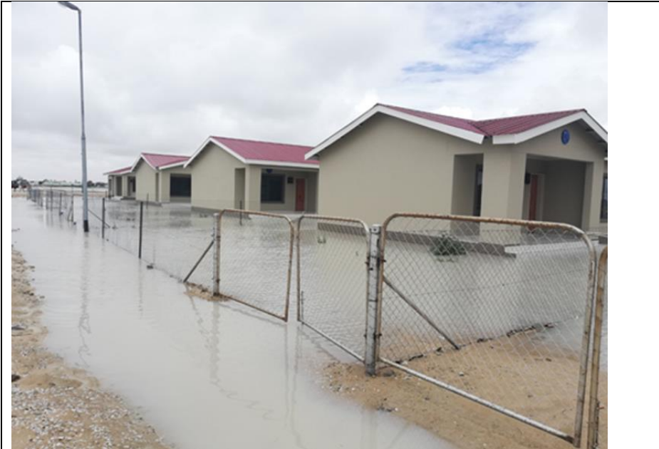
Figure 5.1 Ehenye Flooding- No drainages. Source: https://neweralive.na/posts/oshakati-mayor-to-put-skills-to-the-test
