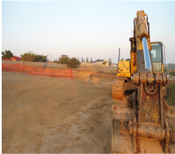
Illustration 11: Water facility being built. In Ward 12 Hibiscus Municipality (permission Ugu District Municipality, Photographer: T. Cele
