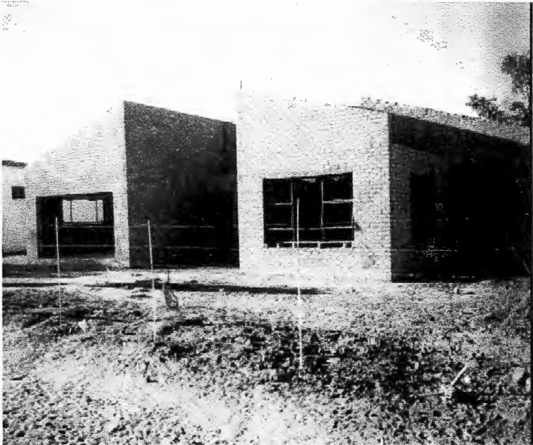
Figure 5.2: A house under construction at Six Hundred-Ramatlabama (Photographed - 25/06/98 )
