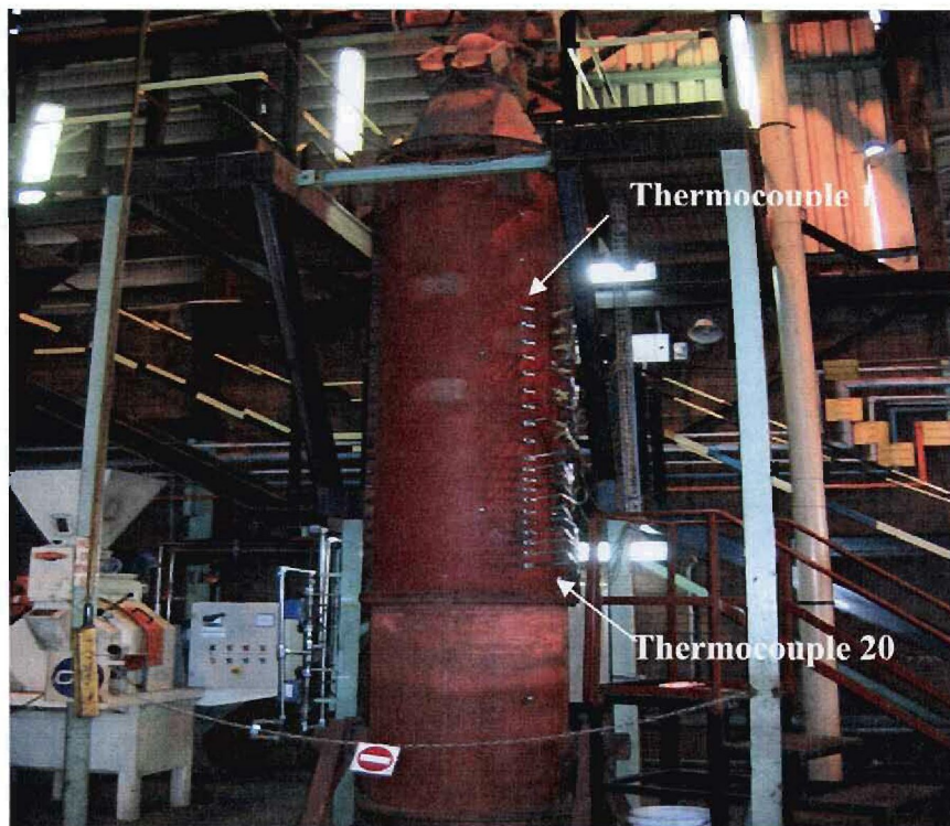
Photograph 2.1: The pipe reactor combustor unit.
