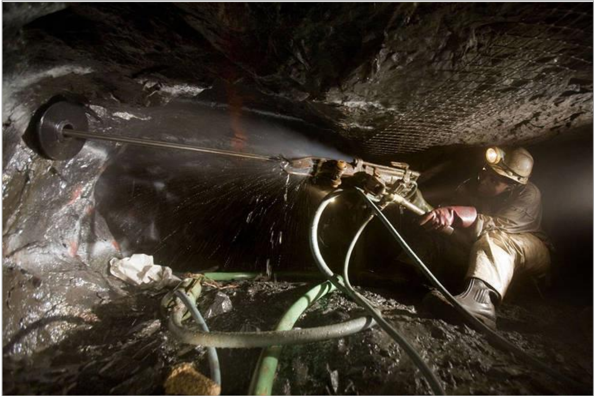
Figure 5: A rock drill operator using a pneumatic drill [18]
