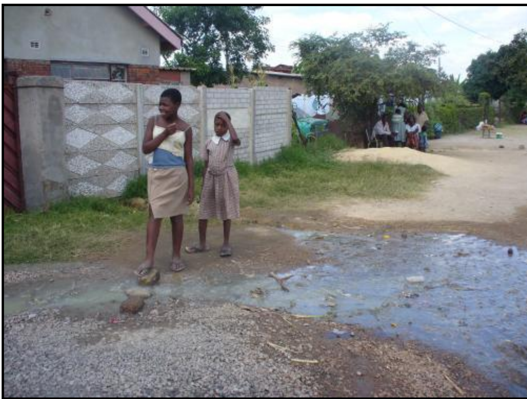
Figure 3.22: Sewerage system failures in Harare
