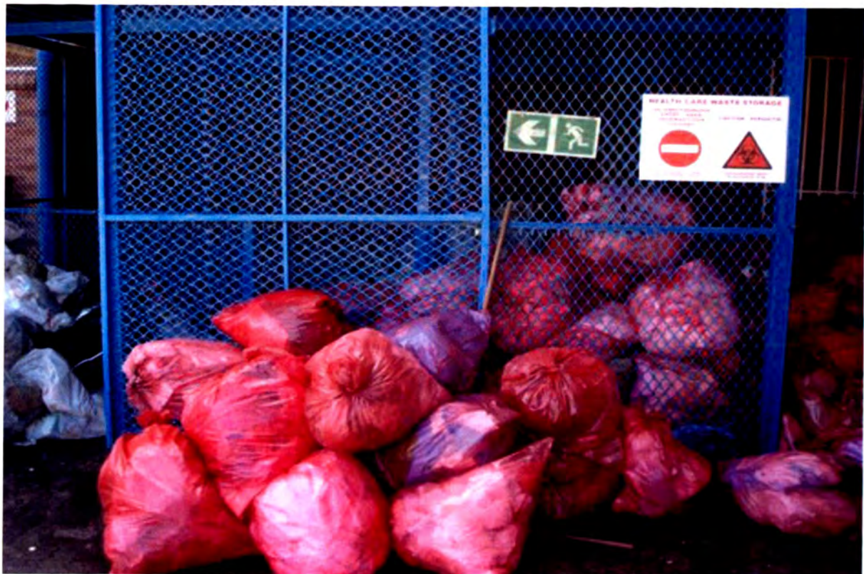
Photograph 3 An Overfilled Temporary Medical Waste Storage Facility (Source: Author 2012)
