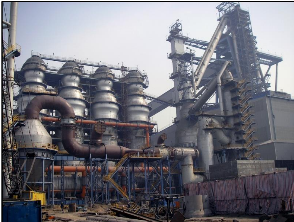
Figure 5: Typical blast furnace with auxiliaries 3
