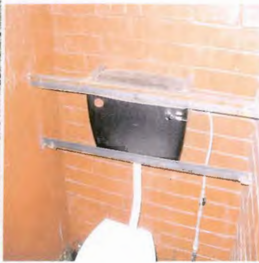
Exhibit 23 Cistern protected against vandalism
